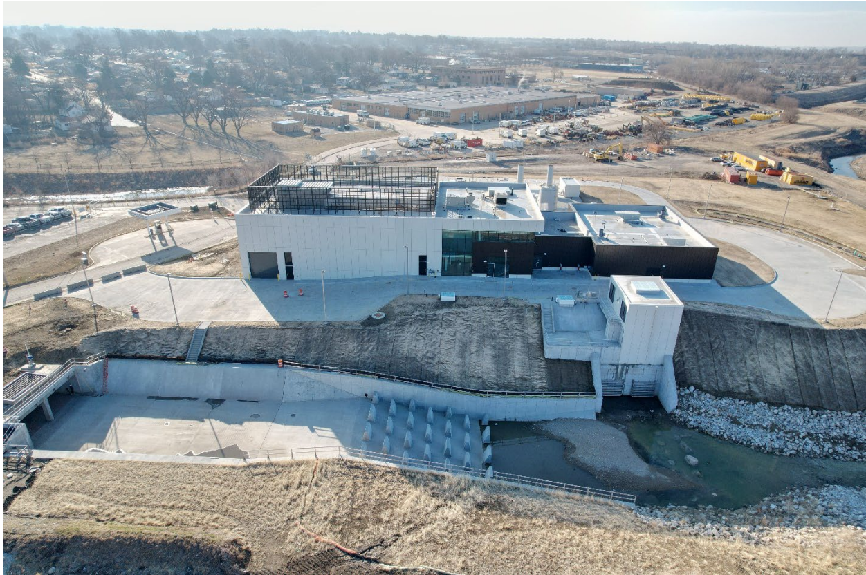
Picture 5 – Construction Progress – March 2023
