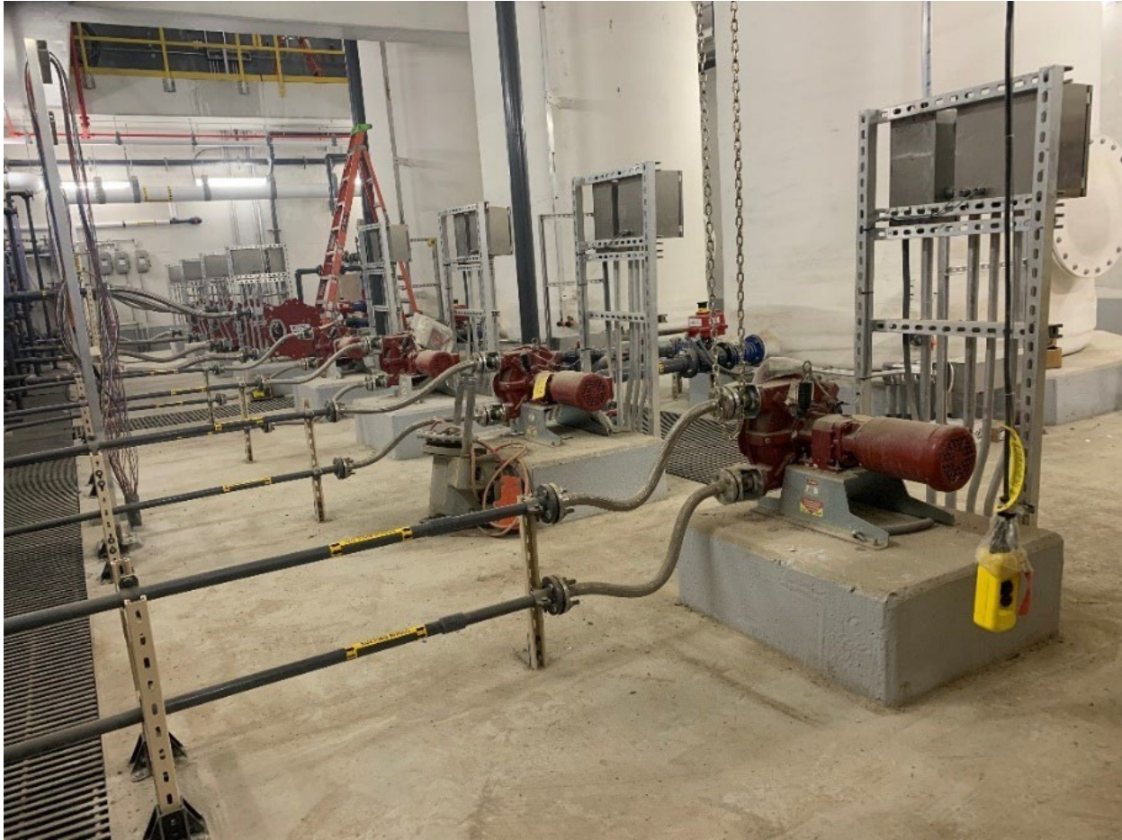
Picture 3 SBS Area of Chemical Building
