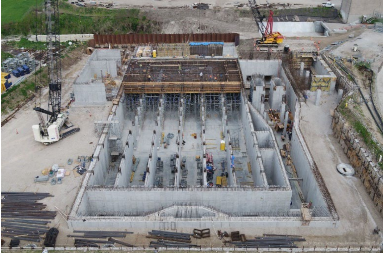
Picture 4 – Construction Progress – April 2021
