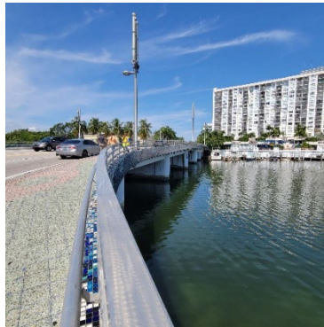
Figure 3. Middle HDD Installation Indian Creek
